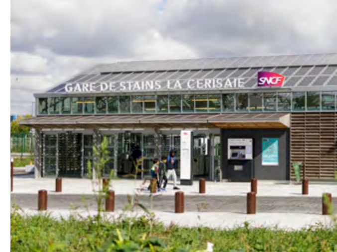
North of Paris, the solar panels at suburban Stains la Ceresaie station provide some of the electricity it needs to operate, and reduce its power bill.
