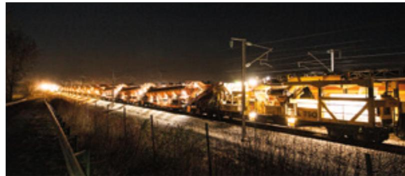
**?** Since 2022, SNCF Réseau has been reusing large amounts of the ballast removed from railway tracks, including from high-speed lines. Currently, up to 65% of the ballast removed during fast-track projects is reused on tracks.
